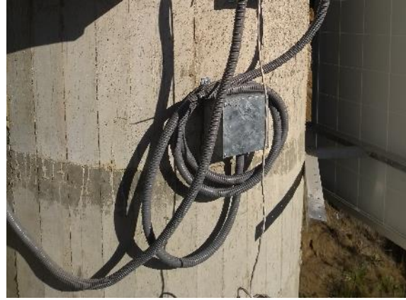
Sensor for monitoring scours, fitted on the reinforced concrete pier
