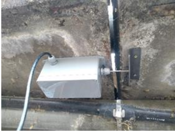
Displacement sensor, installed on an expansion joint
