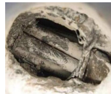
Tendon defect
