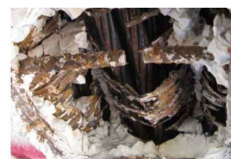
Tendon damage
