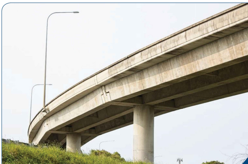
Illustration 6 - Halving joints on cantilever piers supporting Gateway Arterial Flyover (GAF) ©TMR
