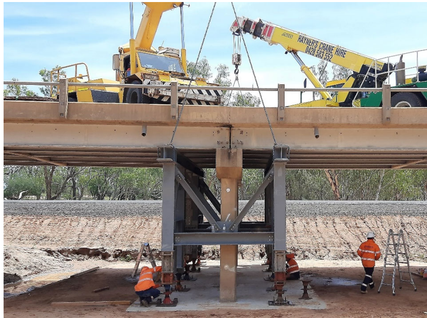
Figure 5 Alice River bridge: Fitting jacking frames to rectify 120mm of pier settlement. (Source: Copyright of the Department of Transport and Main Roads, Queensland, Australia)
