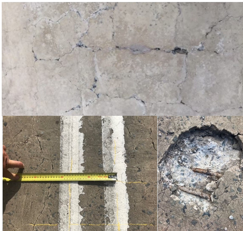
Figure 6 Bee Creek bridge deck slab deterioration
